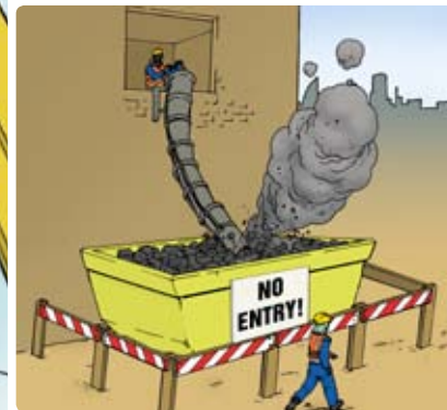
Rubbish chute system with barriers
