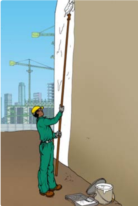
Using long-handled tools instead of a ladder
