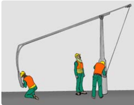
Lowering streetlamp for repair
